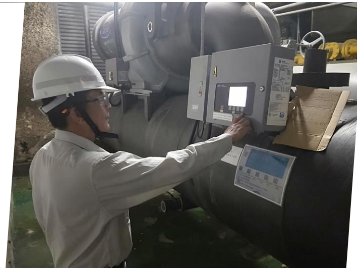
Chiller equipment maintenance
