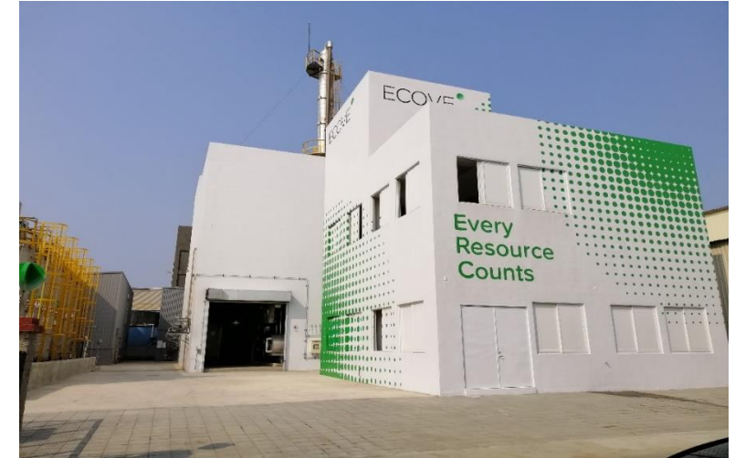
ECOVE SRC Waste Isopropanol Recycling Plant
