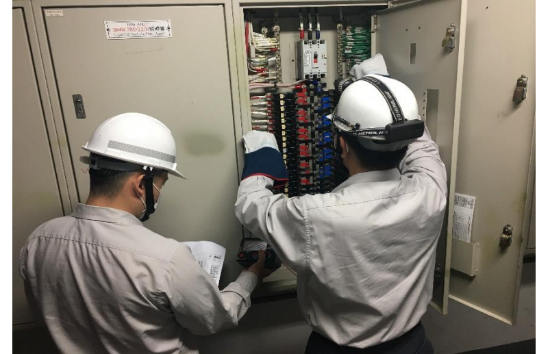
Electrical panel equipment maintenance
