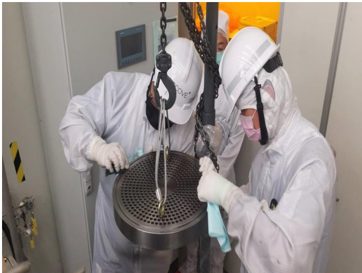
Cleanroom process equipment maintenance
