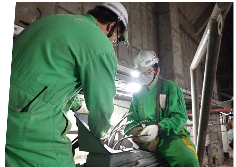
Wind turbine motor replacement
